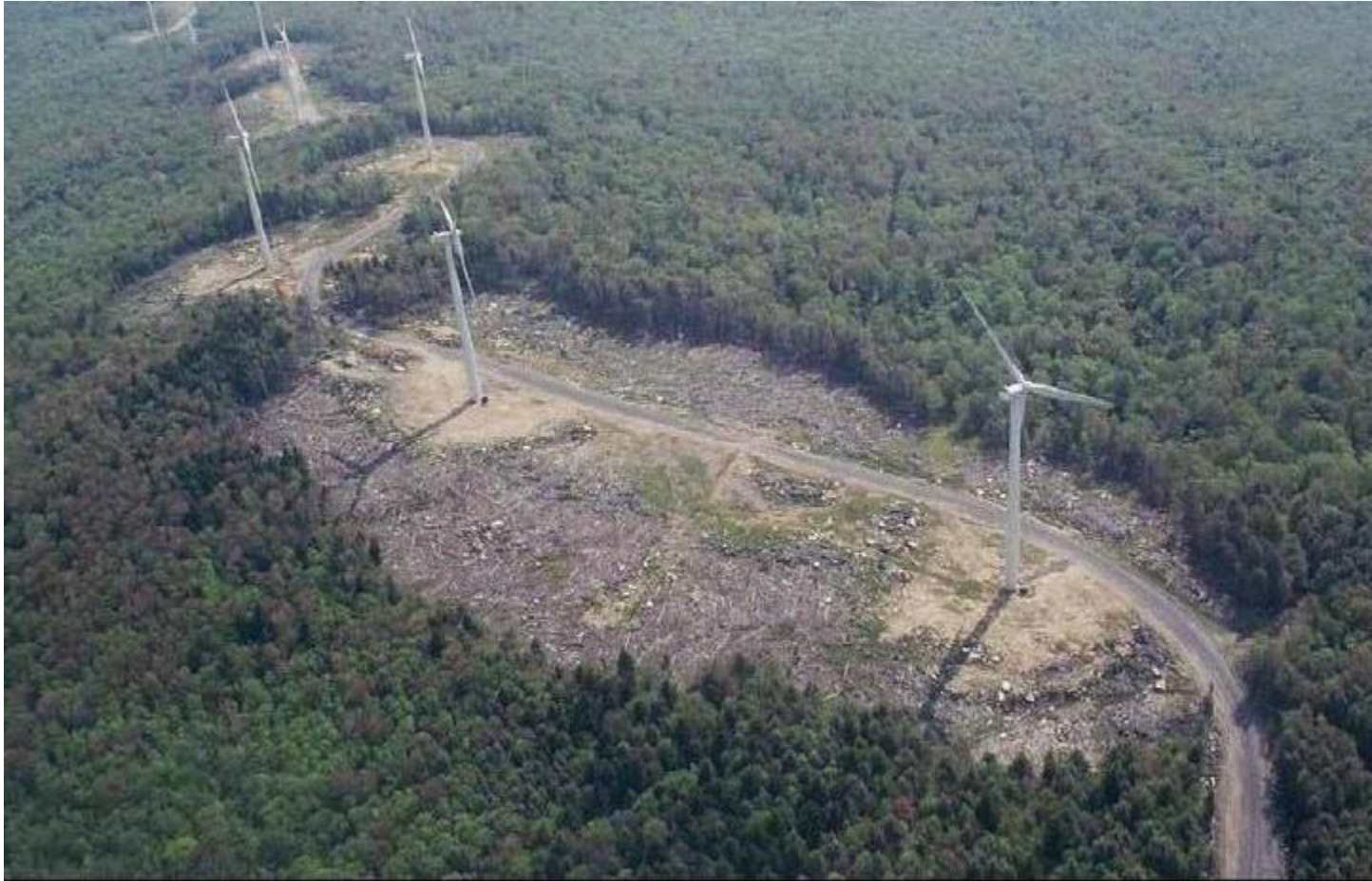
Mountaineer Wind Energy Center, Tucker & Preston Counties, WV
